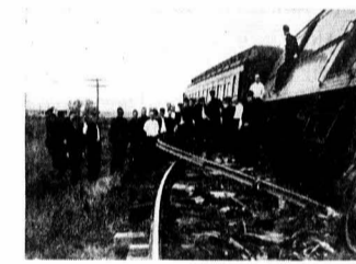
Just after the wreck—the twisted rails bear vivid witness to the speed at which the train left the track.
